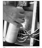
Cleaning the switch box with canned air.
