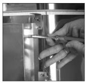
Removing the element cover to gain access to the element connectors. Not all kilns have an element
